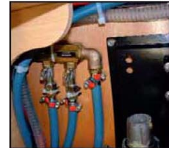
VALVES FOR TANK SELECTION
