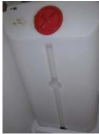
Sewage tank (Landmark 2/3) Capacity: 83 liter
