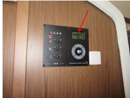
Gauge Location: Passageway
