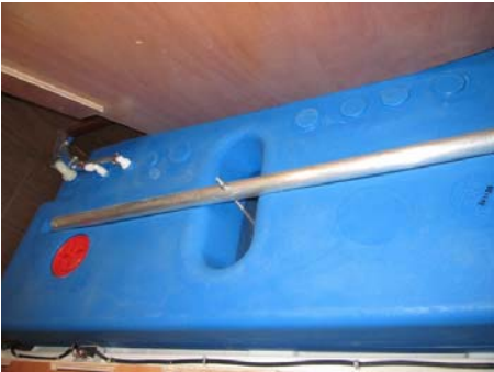
Water tank Location: Aft cabin
